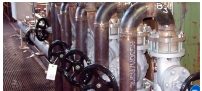
Headers and actuating valves at tuyere level
