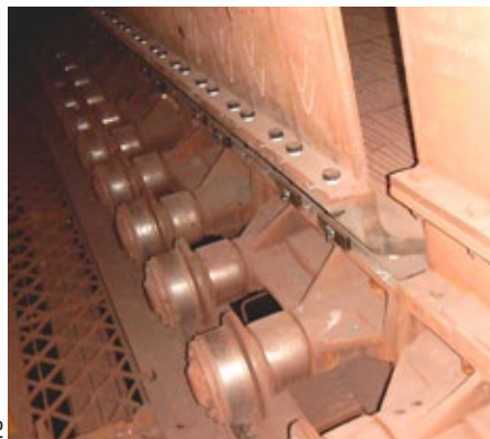
1. Paul Wurth widening in operation
